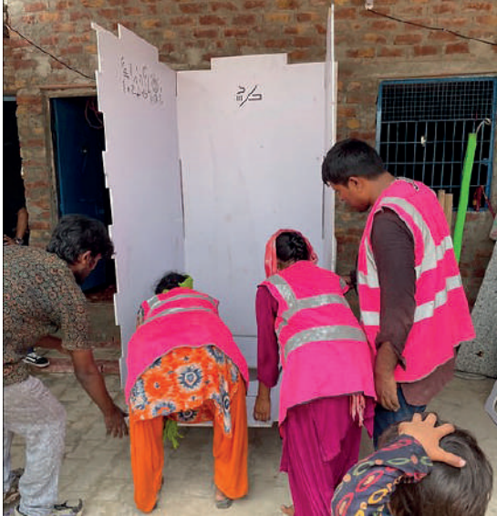
Image 1: Installation of BasicShit toilet at Majnu Ka Tila Refugee camp
