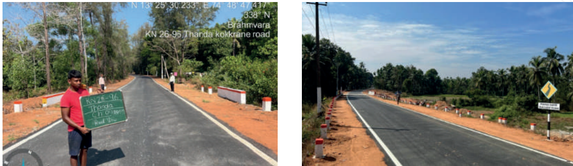
Image 3: Plastic formed Thande Kokkarne Road in Brahmavara Taluk, Udipi District
